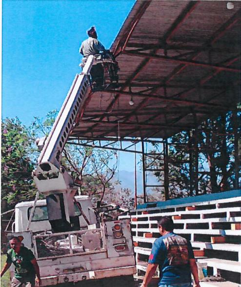
A photograph showing a construction worker perched on a crane's boom, installing a light fixture on the roof of a stadium. Other workers are visible on the ground near the crane. |
