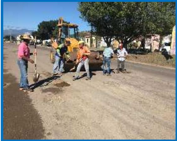
A group of workers in various colored shirts and hats are working on a road. They are using tools to spread a light-colored, granular material (bank material) into a pothole. A yellow tractor is visible in the background.                |
