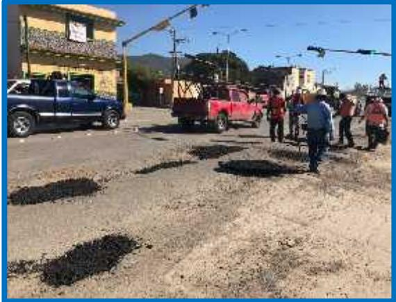
Workers are performing pothole repair on a road. The road surface is dark asphalt, and there are several potholes being filled. A blue pickup truck and a red pickup truck are parked nearby. A traffic light is visible in the background. |
